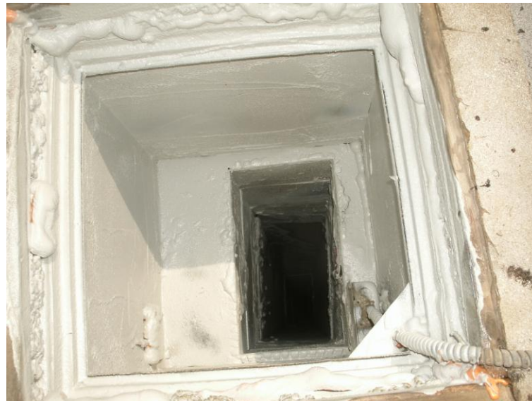
View Under the Fan "After" Sealing
