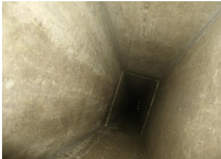
Clean Shaft "After" Cleaning
