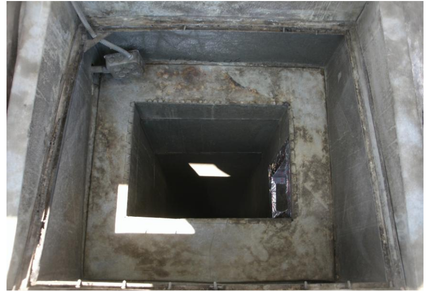
View Under the Fan "Before" Sealing
