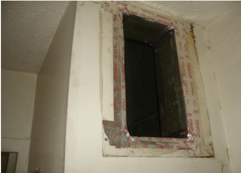
Sealing In & Around Vent Boot
