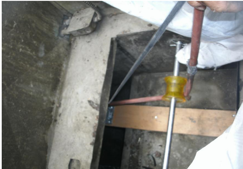
Creative Approach for Cleaning & Sealing Shaft w/ Slightly Longer Lateral
