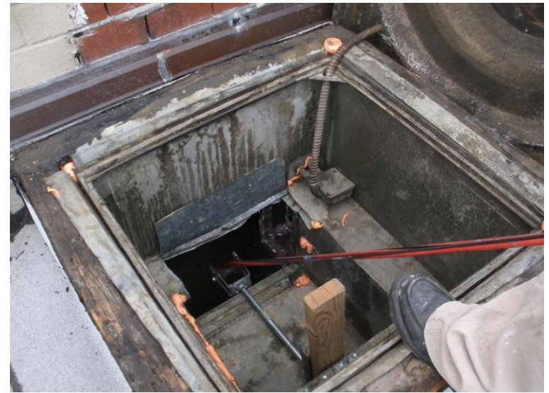
Creative Approach for Cleaning & Sealing Shaft w/ Short Lateral
