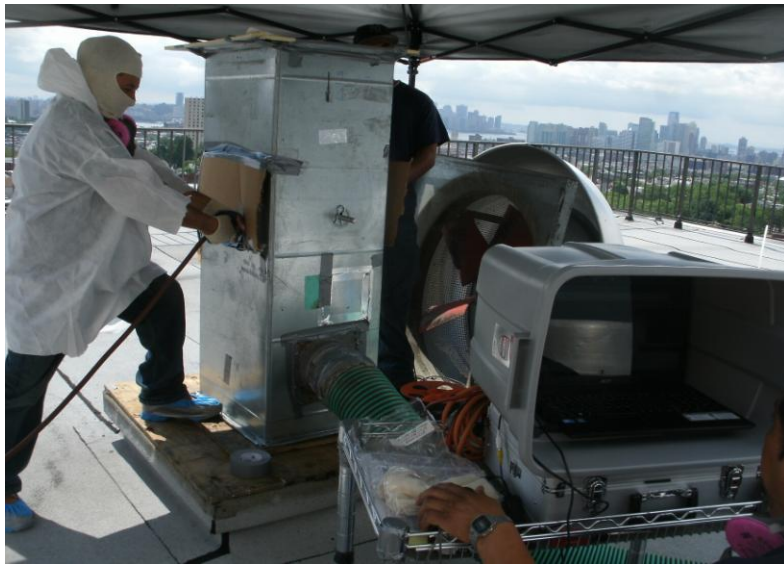
Shaft Cleaning In Progress
