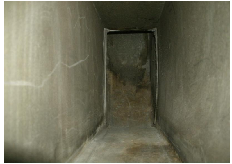
The Same Lateral "After".
