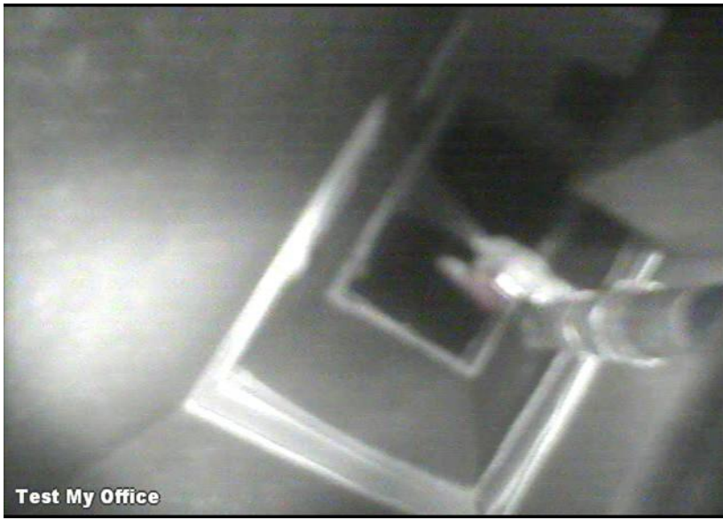
Robotic Sealing of Duct Connection Joints
