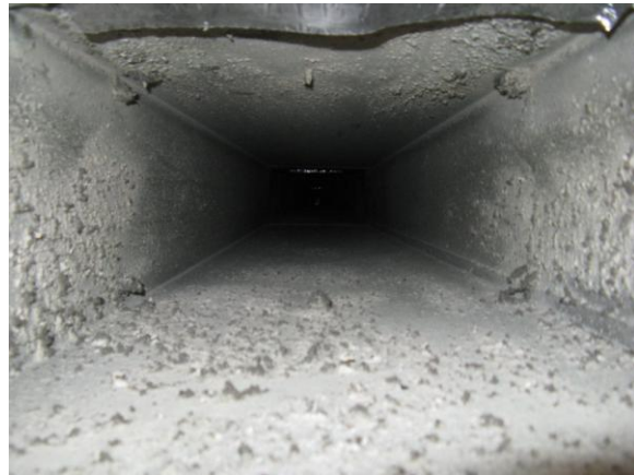
Kitchen riser before cleaning.
