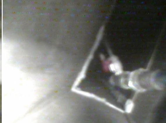
Robot-Controlled Spray Head Applying Mastic
