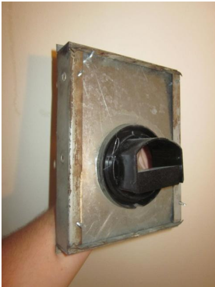
CAR Damper Assembly For Bathroom before Installation
