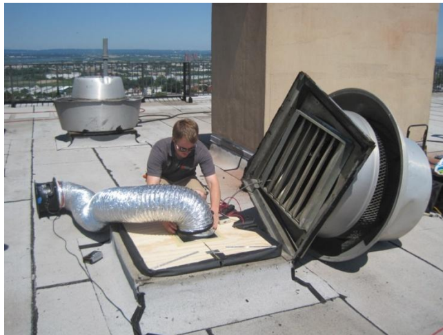
Duct Leakage Test in Progress
